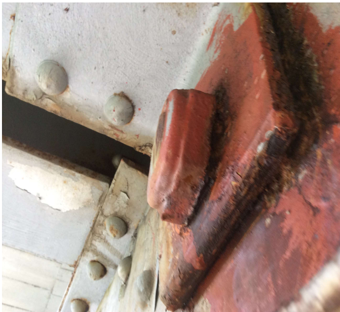
PHOTO 4 Description U-42 right pin has out of plane bending.
