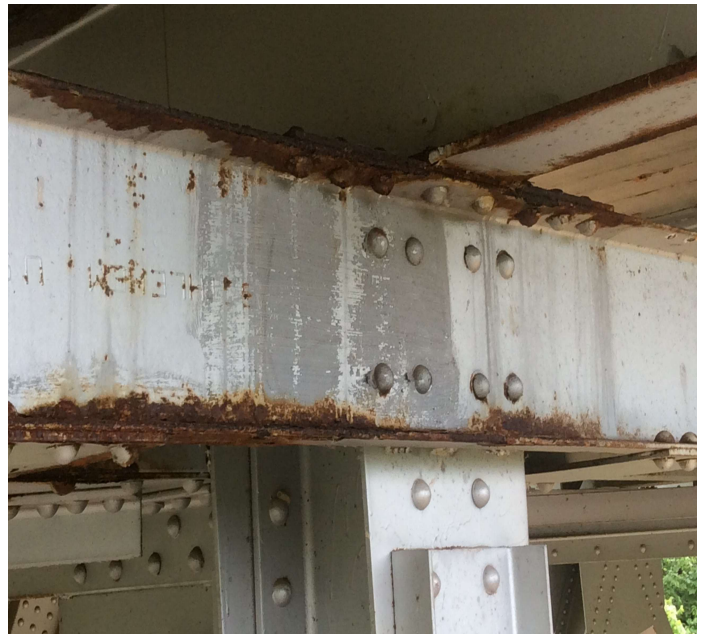
PHOTO 2 Description U-29 right active corrosion to top cord with flaking rust.
