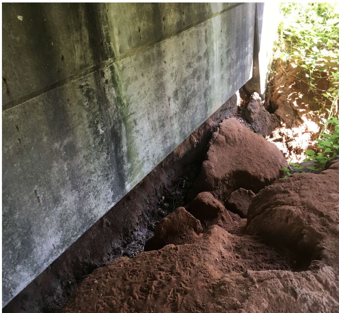
PHOTO 1 Description Embankment erosion at abutment #1 that extends under the web wall of the abutment.
