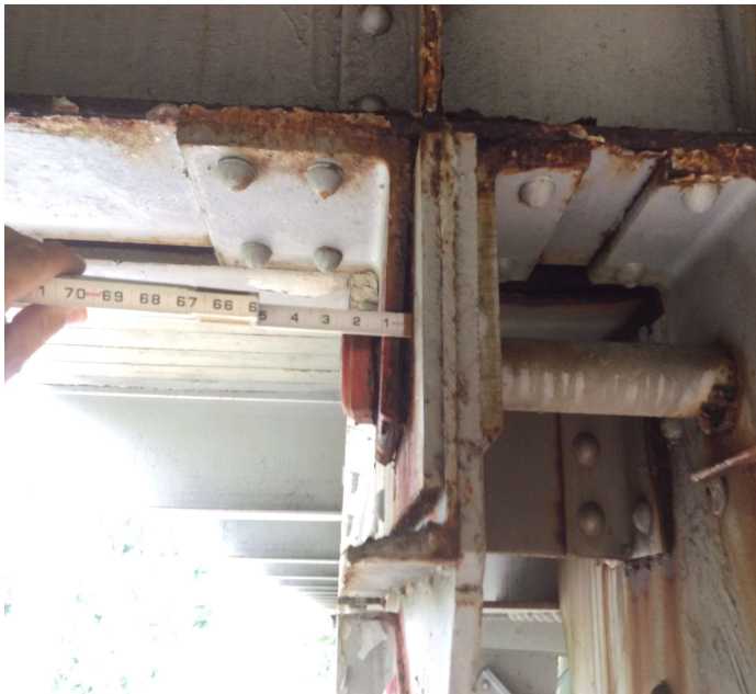
PHOTO 3 Description U-42 right pack rust minor out of plane bending to pin and pin connection.
