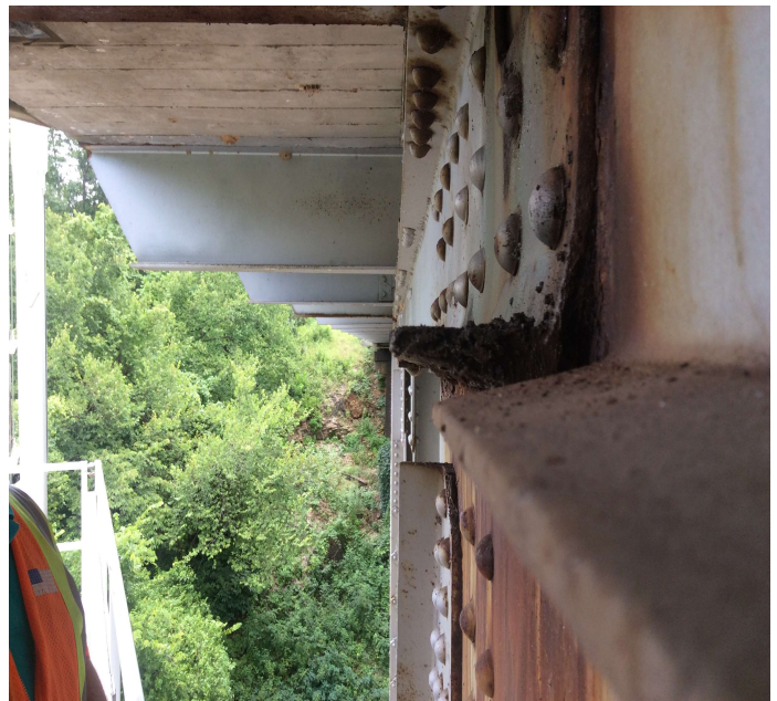
PHOTO 6 Description U-26 left top cord pack rust with out of plane bending.
