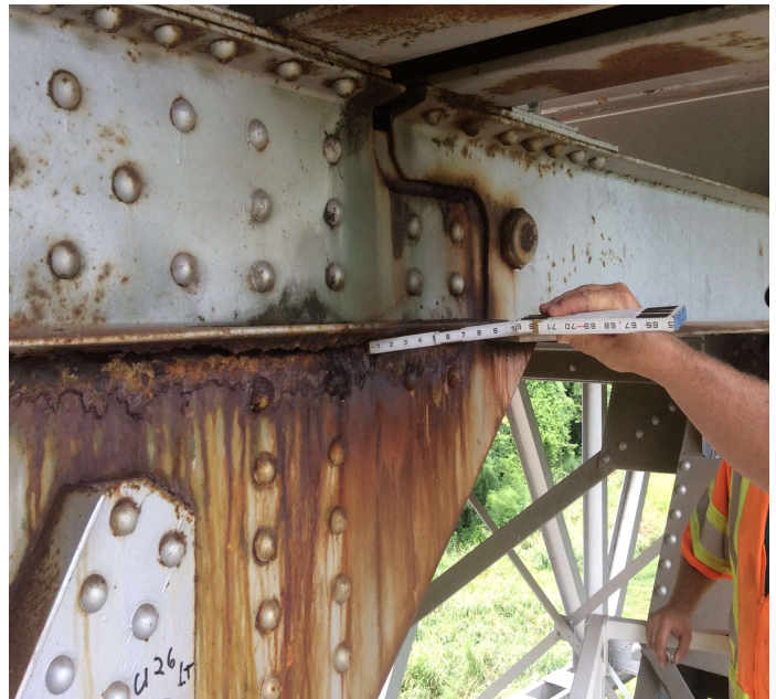
PHOTO 5 Description U-26 left pack rust with measurable section loss top cord and gusset plate.
