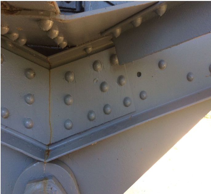
PHOTO 1 Description Rivet sheared off at the interior bottom chord connection at L 15 right truss.
