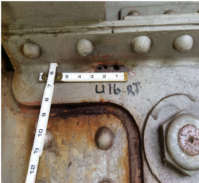
PHOTO 1 Description U-16 right holes rusted through web section.
